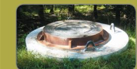
What appears to be a manhole is actually a stormwater treatment unit. Units such as this one use a settling tank to filter contaminants from runoff. Runoff is piped into an upper chamber and is then diverted to a lower settling chamber, where sediment settles to the bottom, and floatable pollutants, such as oil and grease, rise to the top of the chamber. After contaminants are separated from runoff, water is displaced up through a riser pipe and is discharged to the storm sewer system.
