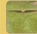
A grassed swale can be used in place of a storm sewer pipe to convey runoff from an area. Vegetation planted in the swale enhances infiltration of runoff into the soil and aids with slowing runoff which allows particles to settle out. Swales may be constructed with a subsoil mix that improves infiltration. The swale at this site incorporates such a mix.
